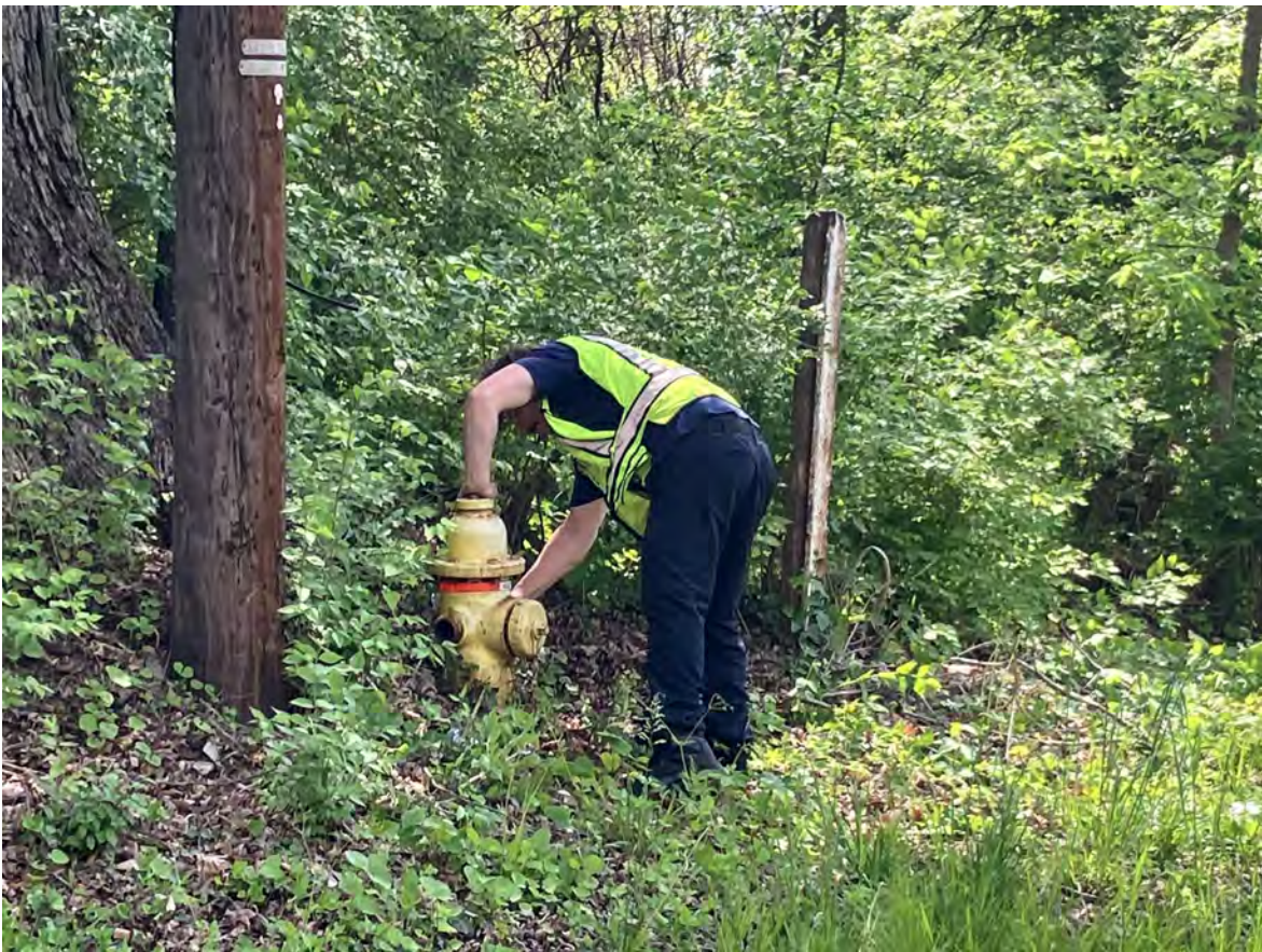
One of the duties of the on-duty crew is to inspect fire hydrants to ensure they are operation in the event of a fire. Here, FF/EMT Tim Linz is seen inspecting a hydrant in Columbia Township in the spring of 2025.
