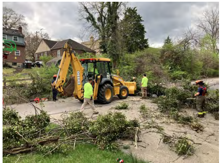
The crew of Quint 89 and Golf Manor's service department worked to clear a tree that was blocking the road on April 4, 2025.
